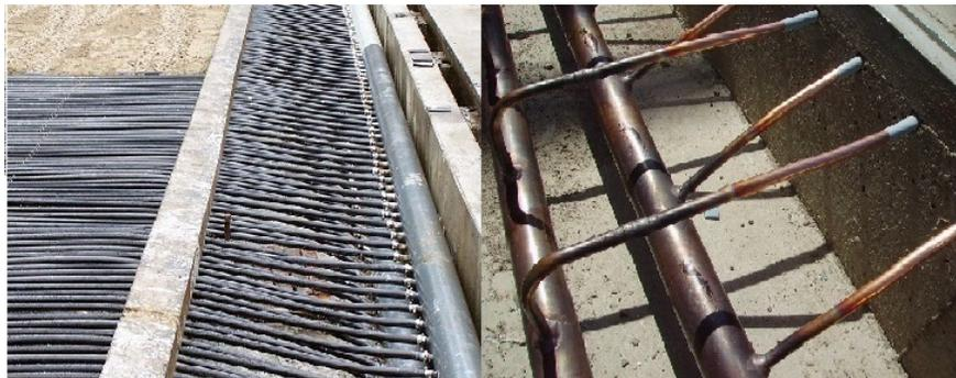
Figure 18: Piping arrangement in distribution system (Katrineholm ice rink project 2006)
